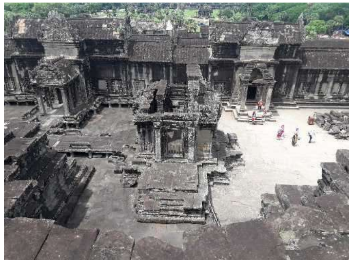
Fig. 11. In this view from near the top of Angkor Wat, the fallen stones are just visible on the right.
