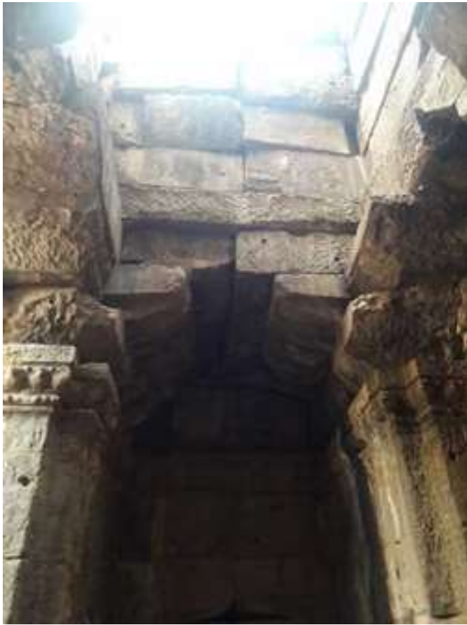
Fig. 3. The well-planned cutting and fitting of stones by ancient workmen are evident at a construction at Sambor Prei Kuk (6 th to 9 th century). The visible blocks can be scanned and input for learning by AI and Machine learning.
