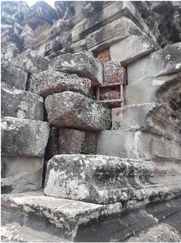
Fig. 12. The well-planned cutting and fitting of stones by ancient workmen in the Angkor Wat, that has allowed its standing for 900 years.
