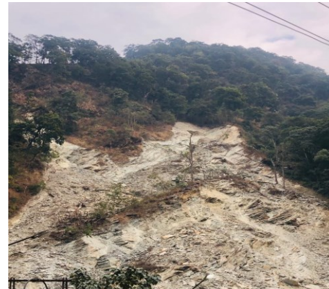
Fig. 1. Debris during a landslide.
