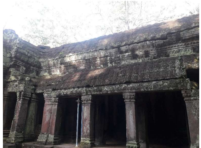
Fig. 19. The reconstructed structure from figure 19, with stones randomly placed, with modern added stones, and supporting modern beams and pillars.
