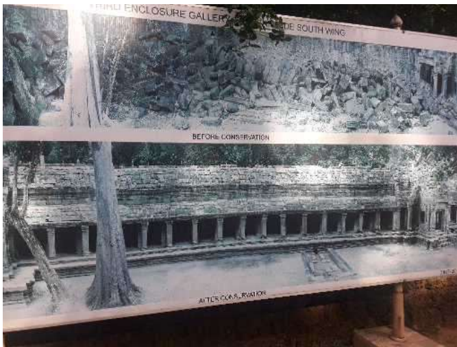
Fig. 18. In this picture at the site, reconstruction of the Bayon temple was attempted with supporting concrete, and the building blocks were completely moved around.
