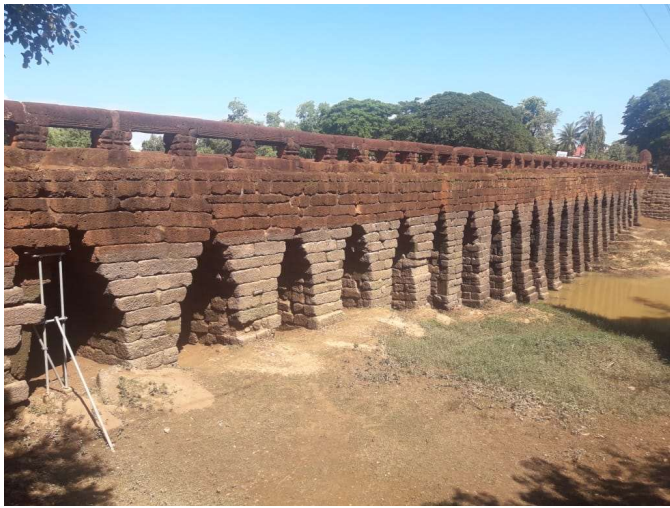
Fig. 1. The well-fitting stones of the still-operational Kampong Kdei Bridge in Cambodia from 1186 AD, that has withstood the worst floods in the last 800 years. The visible structure can be scanned and learned by AI and Machine learning.
